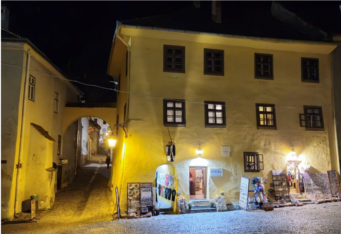
House on Piața Cetății in Sighișoara where Vlad Drăculea was born in 1431 (photo: Dénes Harai, 29 October 2024)
