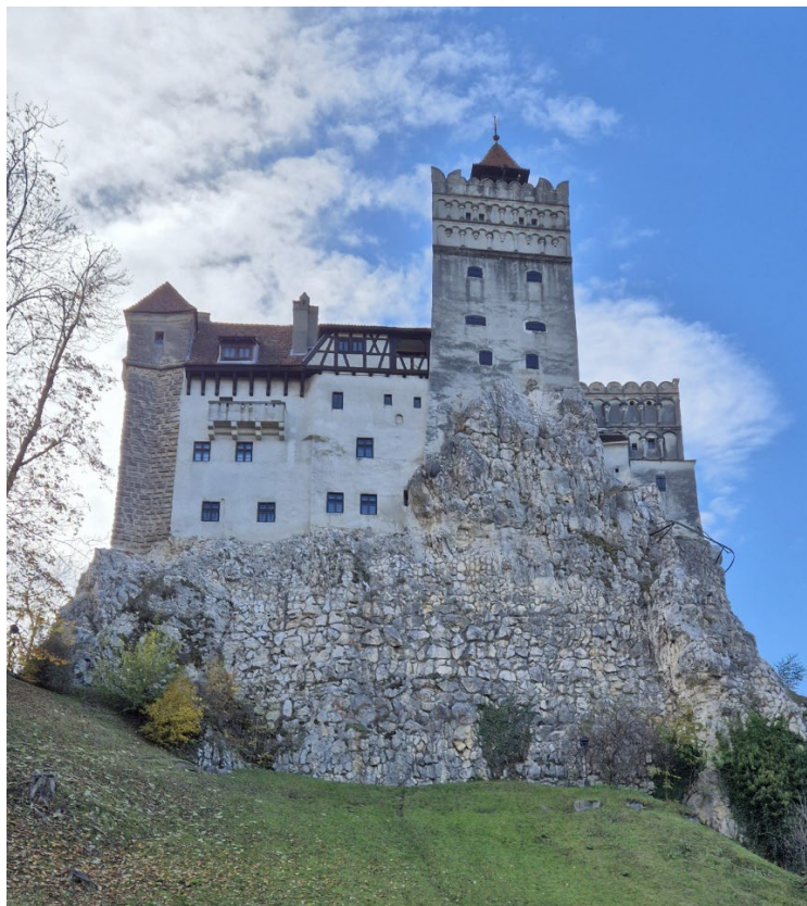
Northern façade of Bran Castle (photo: Dénes Harai, 30 October 2024)
