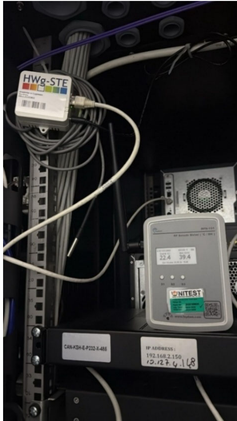
Figure 8. 11. Redundant temperature and humidity monitoring via wired IP and wireless RF sensors
